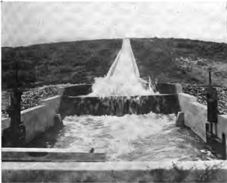
FIG. 128.—Concrete Chute and Stilling Basin, Boise Valley, Idaho.
